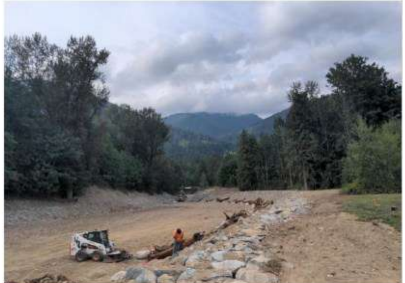
Final touches on sediment basin
